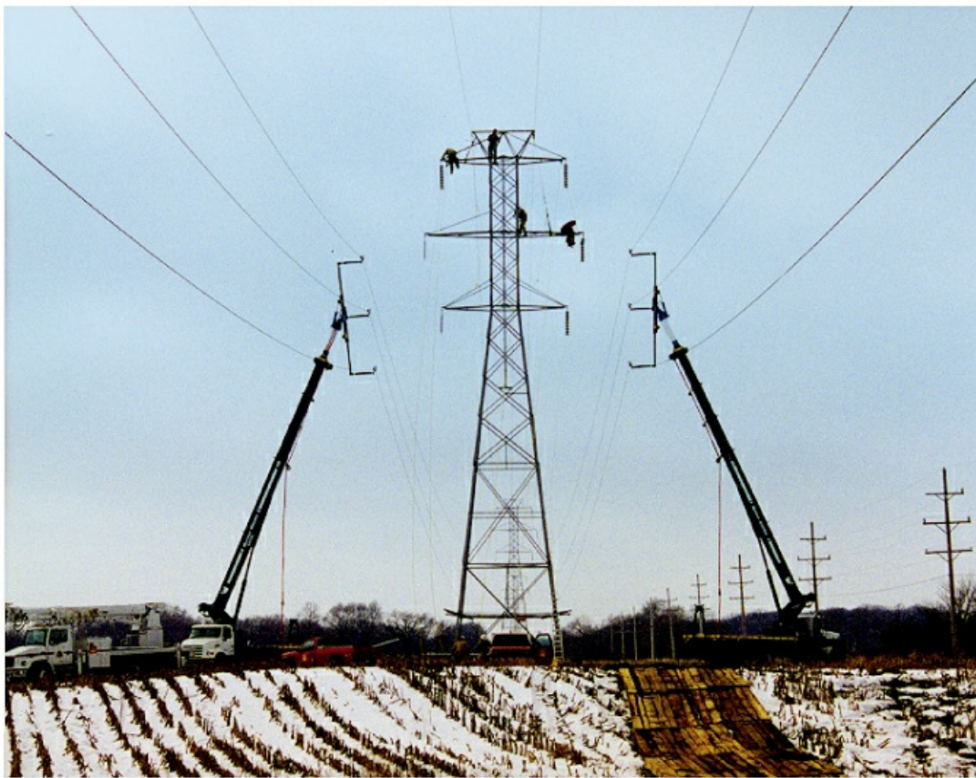
Energized transmission lines removed from steel structure by Linemaster® robotic arm to provide a safe work environment for employees.
